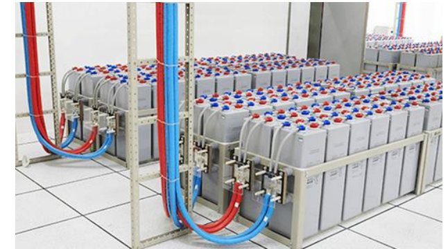
Inside view of large containers Each battery pack contains a BPMS sensor
