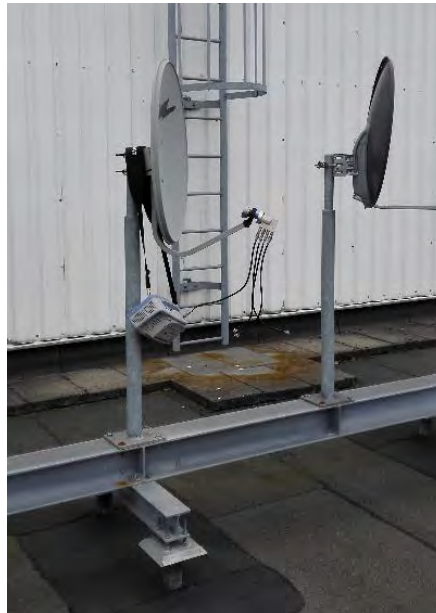
Figure 37 Live signal test setup
